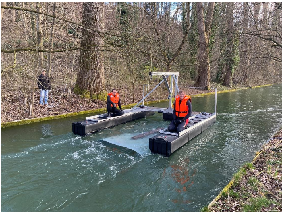
Figure 2: The Energyfish can be installed and commissioned within a few hours. © Energyminer GmbH
